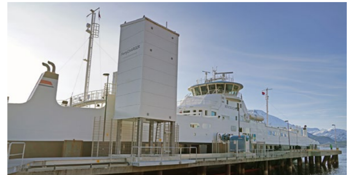
Charging towers quickly supply the ferries with a large amount of electricity. In just one minute, they can supply a ferry with the same amount of electricity as an average household uses in one day.
